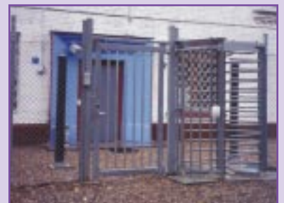
Physical Protection Upgrades in Belarus
