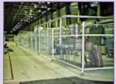
Physical Protection Upgrades at Elektrostal
