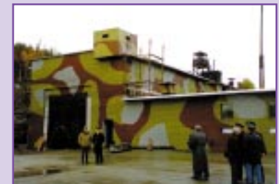
Annex to Northern Fleet Fresh Fuel Storage Site
