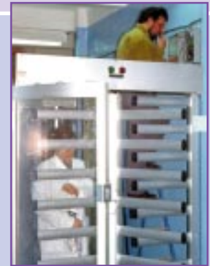
Personnel Access Control (mantrap) at Arzamas-16
